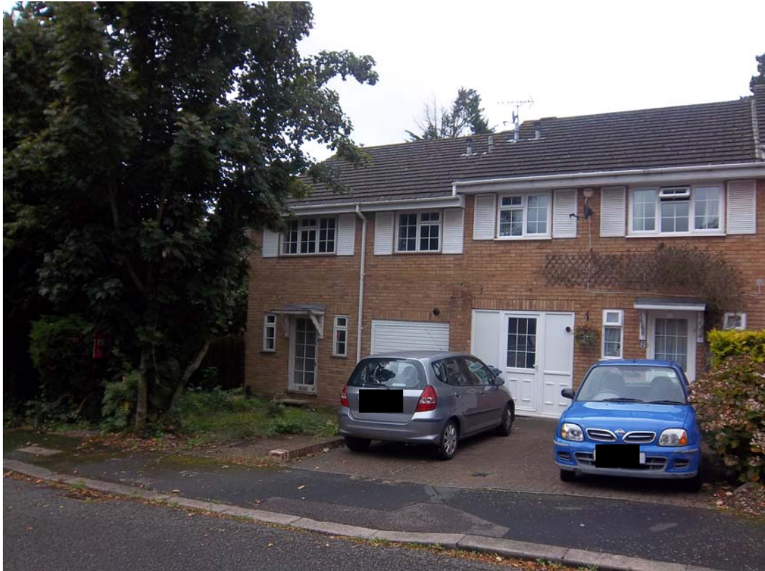
View of no. 2 which has two parking spaces at the front
