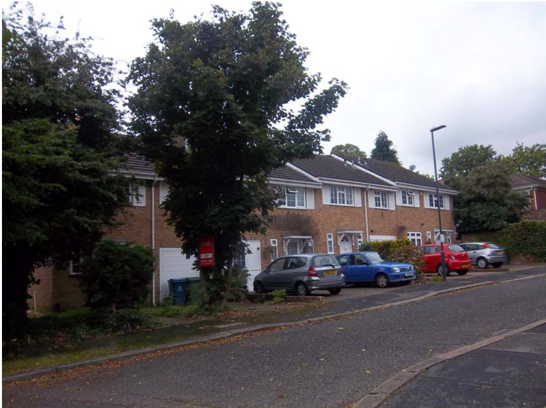
View of the terrace Nos. 1, 2, 3 and 4 Lorraine Park (left to right)
