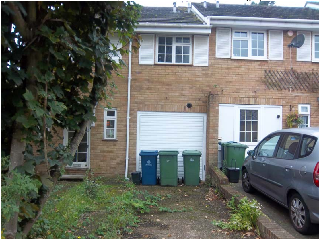
Existing bin storage located at the front of the property
